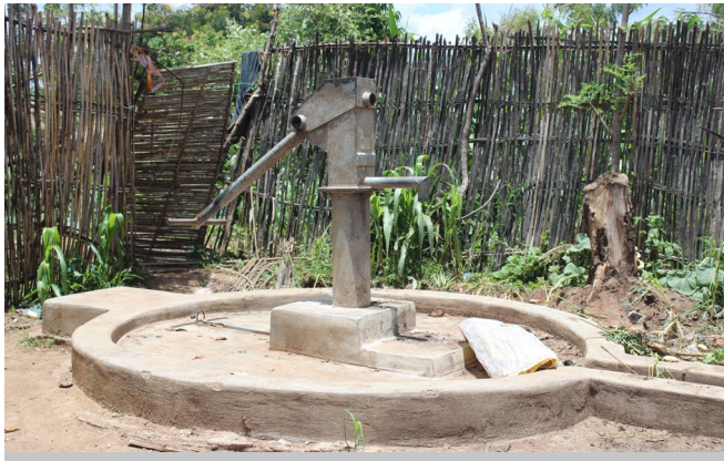
Example of a village well in rural regions of Southern Africa – these wells often supply contaminated water. ©Fraunhofer IST, Jan Gäbler
