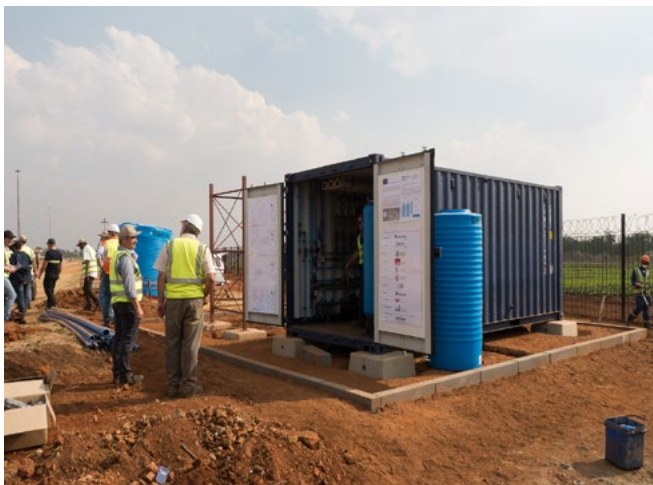
Installing the water purification system. © Fraunhofer IST
